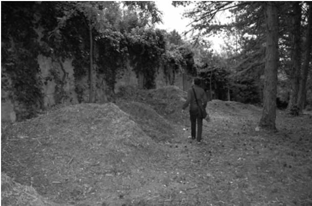
Fig. 1. Boundary garden wall overgrown by ivy, with chopped plant material (Photo: J. J. Purger).
